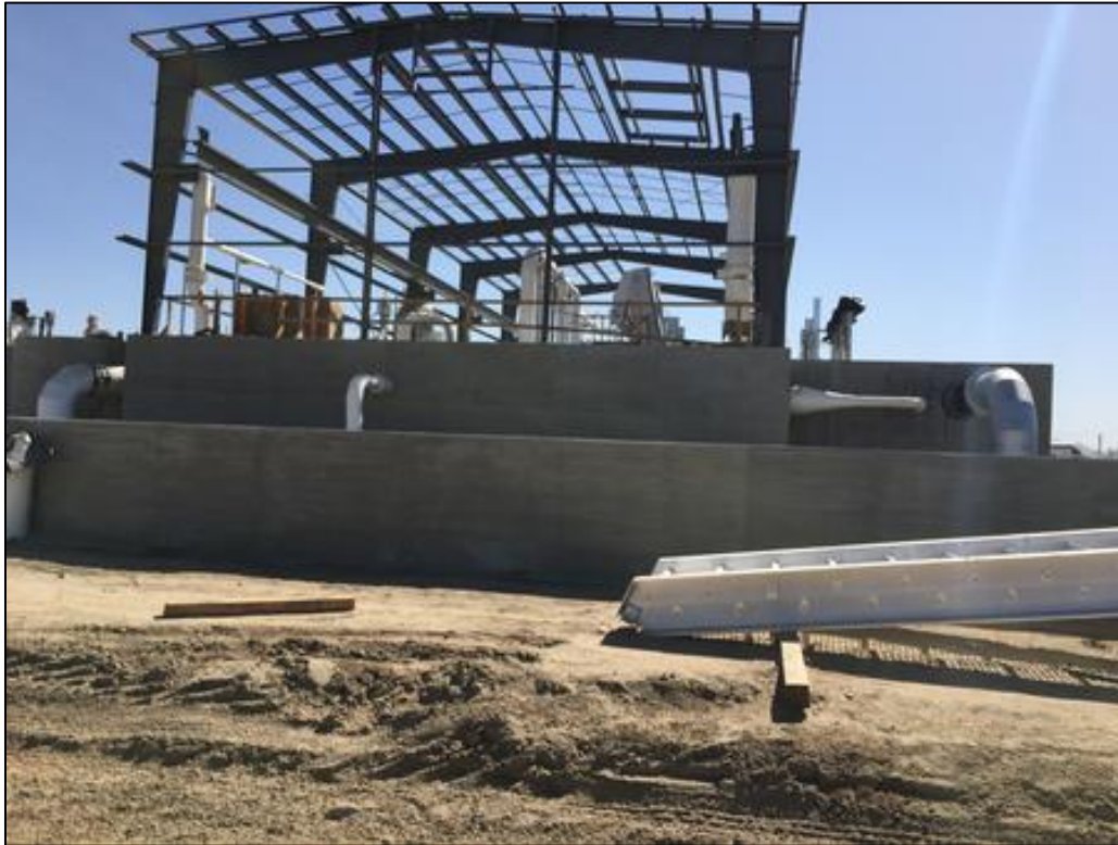
Headworks Building steel frame - view from north
