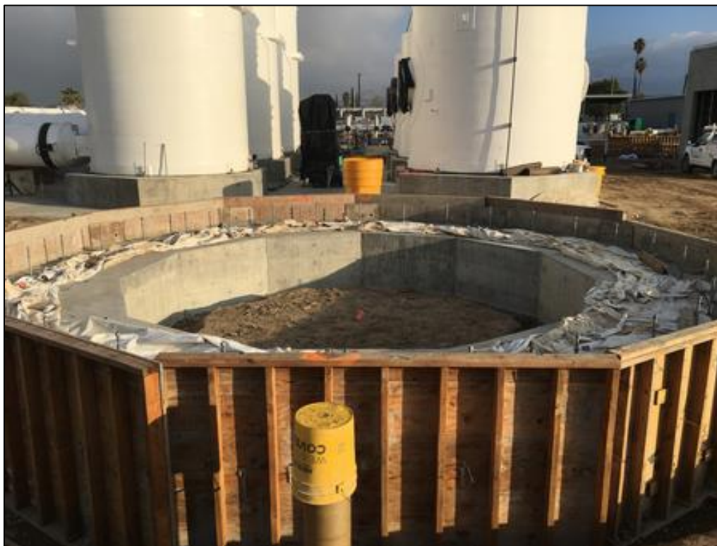
Ring footing for filtrate storage steel tank
