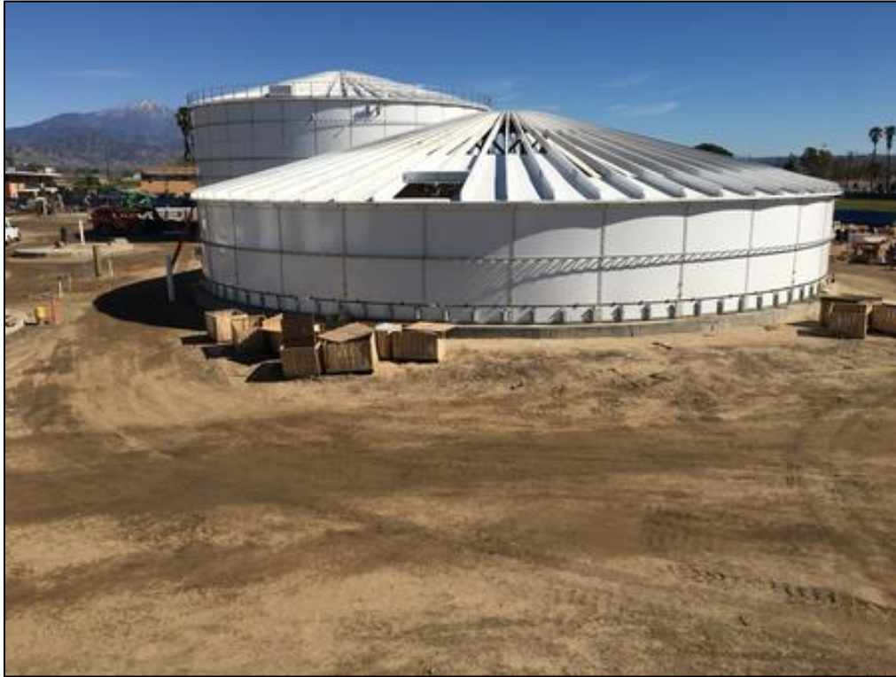
Both Digesters under construction
