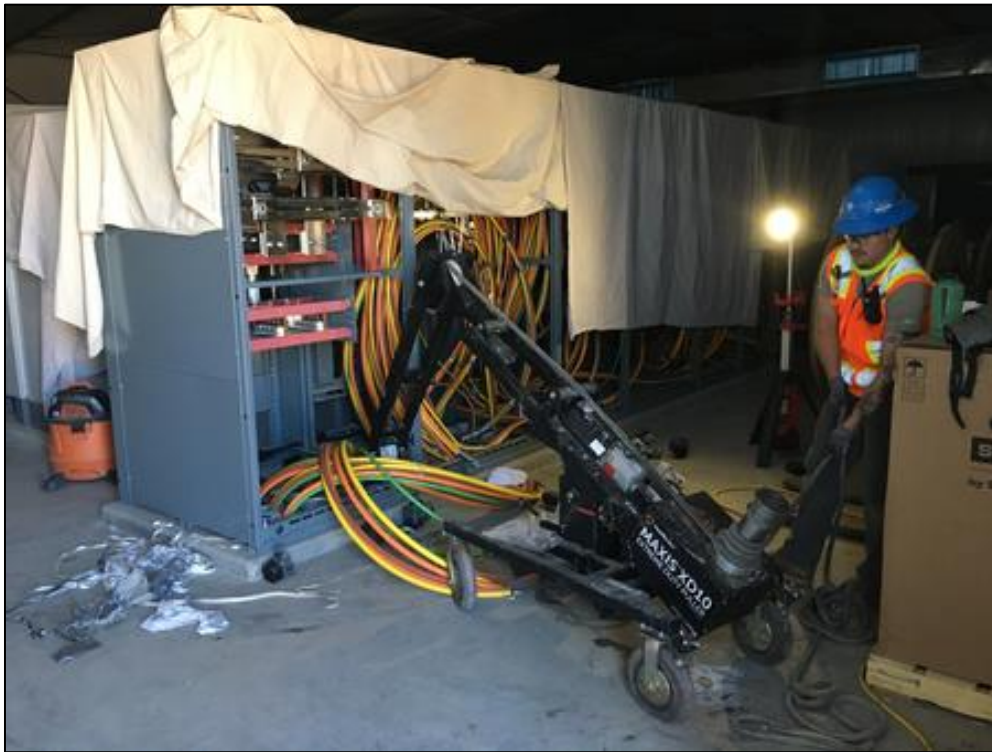
Wiring being pulled in Main Electrical Building
