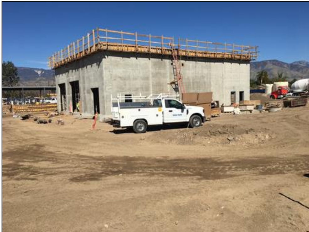
Lower-level walls of Biosolids Building
