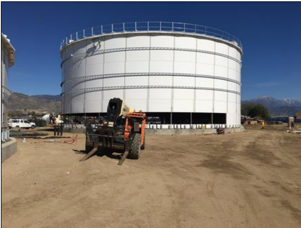
Vertical lift and wall plate installation on east digester
